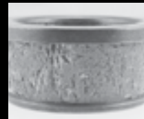
Severe peeling and spalling from heavy loads
