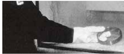
Thermostatically-controlled freezer units aid in the installation of tight-fitted cups in hubs.
