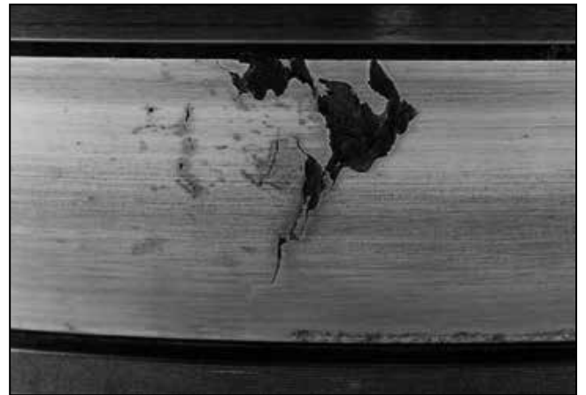
Fig. 170. Point surface origin spalling (PSO).
