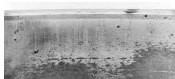
Peeling on raceway
