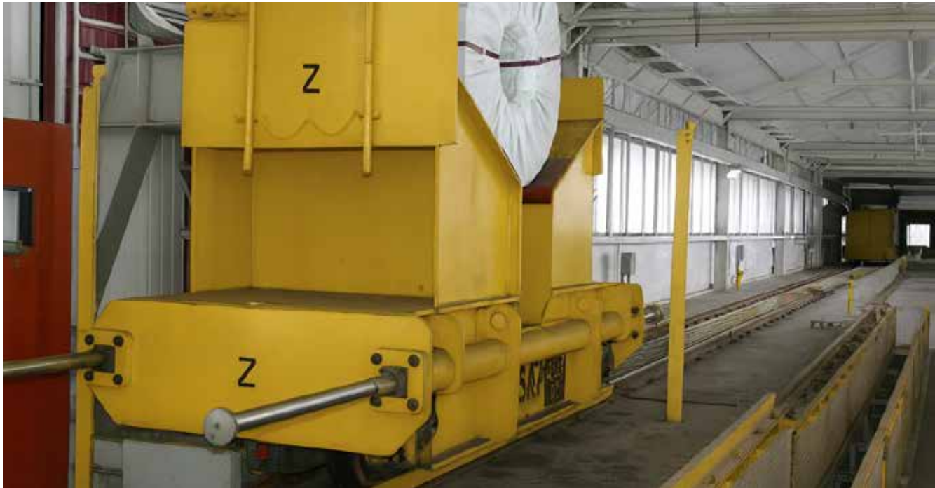
Fig. 18 Coil transfer car equipped with AP bearings on axles
