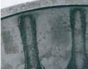
**Staining:** Surface stain with no significant corrosion from moisture.
