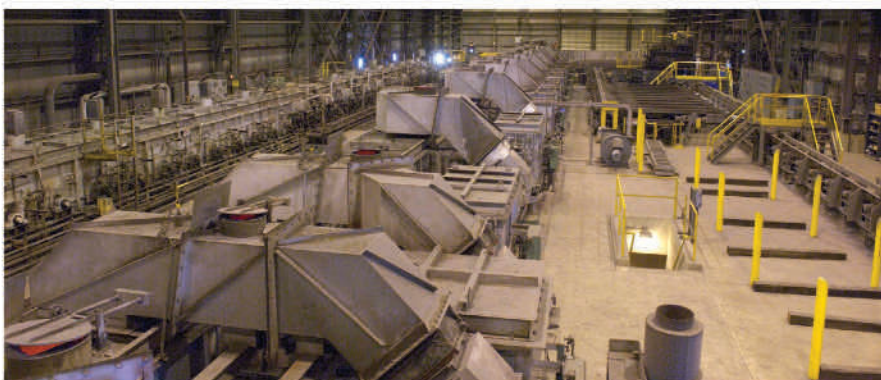
Austenitizing/Tempering Furnace/Straightener at CTF Facility.
